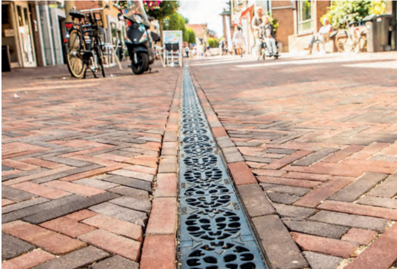
CITY CENTER Baarn, Netherlands (designed by Marlies van Diest)
